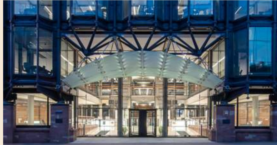
Bracken House Grade II* listed conversion into the The Financial Times HQ, EC4
