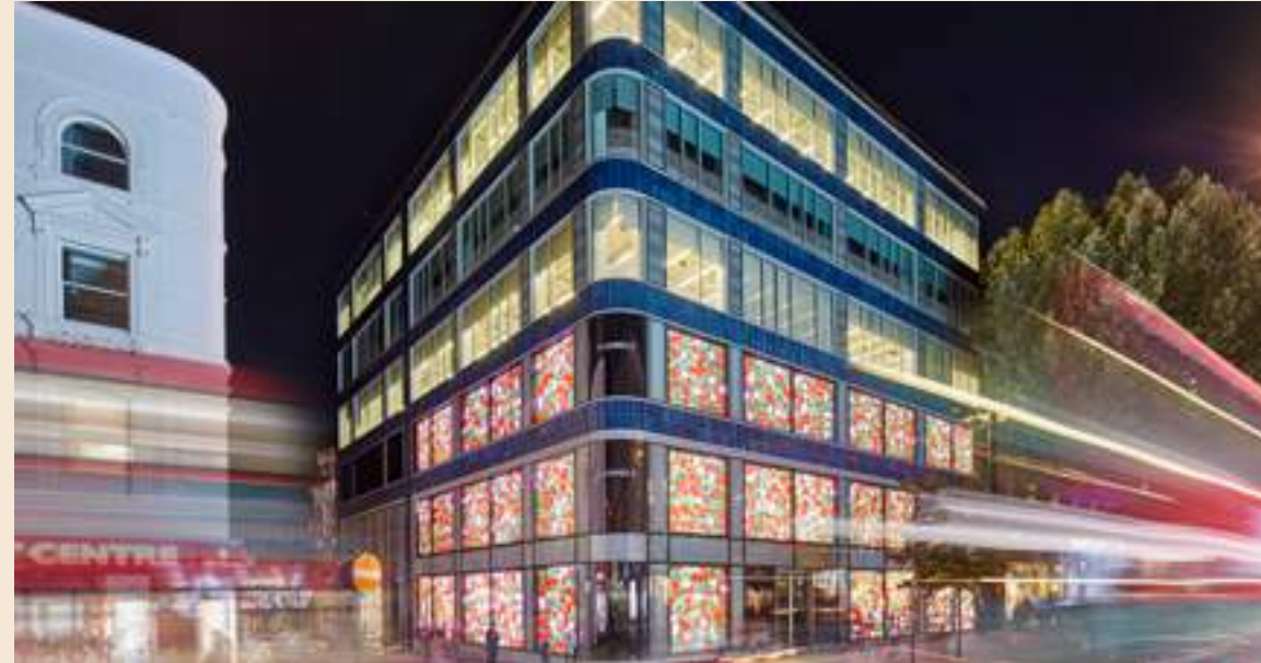
Academy House Refurbishment and re-cladding of Academy House, W1
